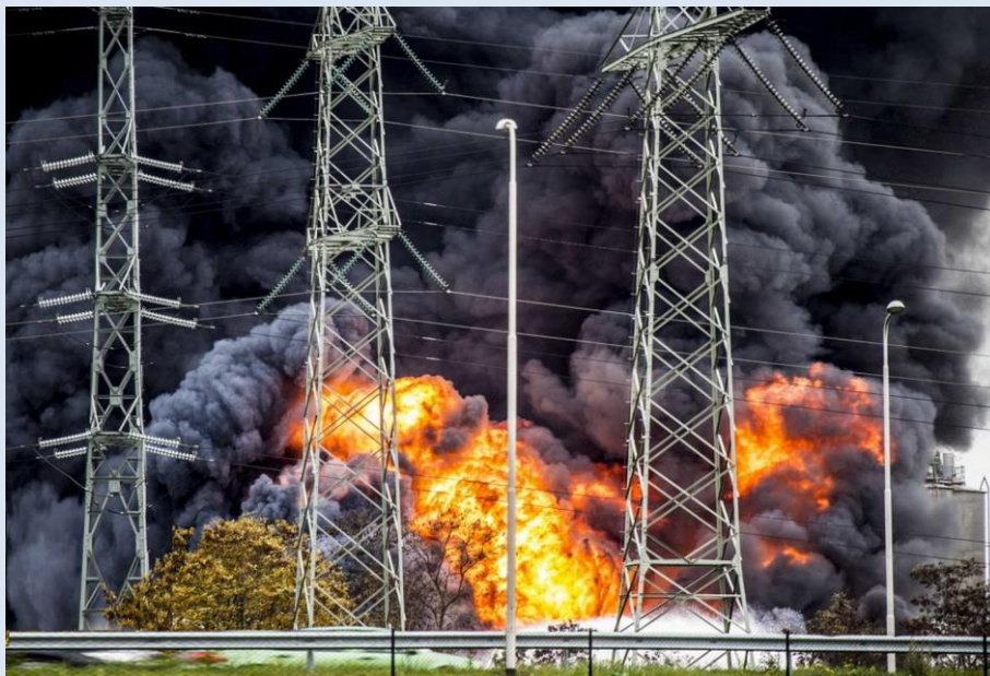
Brand op Chemelot terrein, 9 november 2015 [35]
